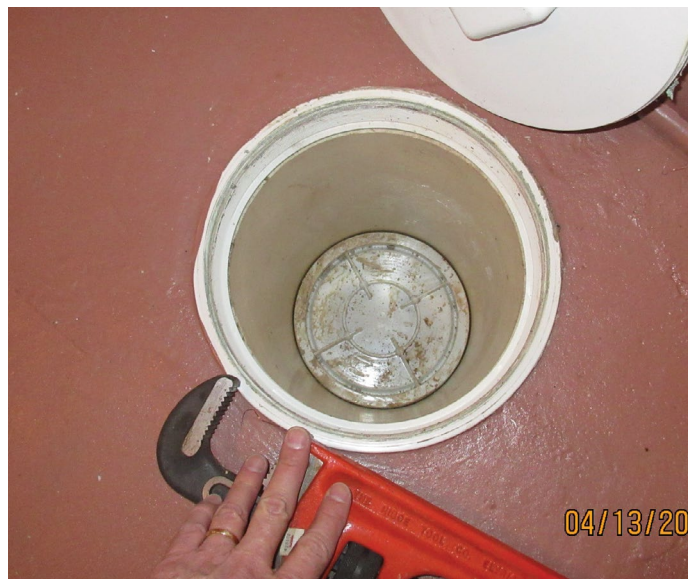
Photo 1. Sewer check valve access.
