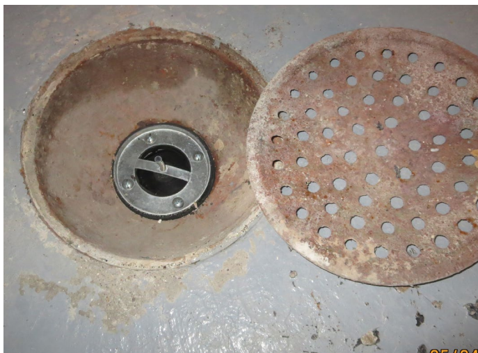
Photo 2. Floating ball check valve.
